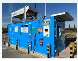
All-in-One is a CNG filling station inside a metal enclosure available for full operation. It includes the following components:
